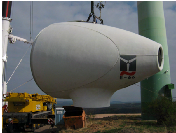
Figure 1: Retirer la salle des machines
